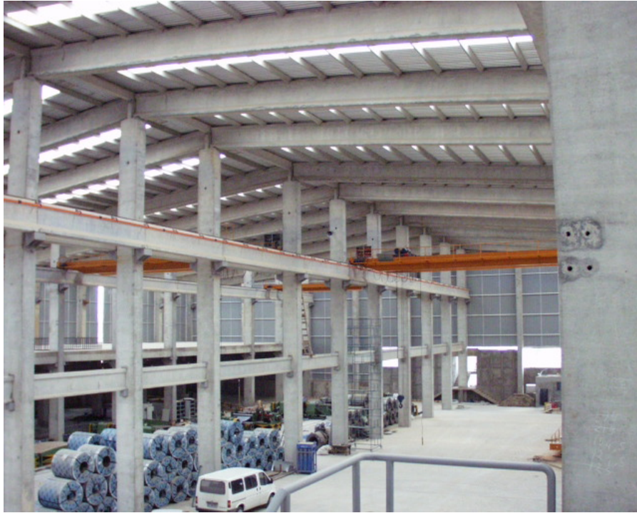
Figure 1.7 Interior Photograph of a Multi-Story Precast Building
