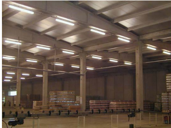
Figure 1.4 Interior Photograph of a One-Story Precast Building
