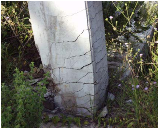
Figure 1.9 Damage Near the Base of Columns
