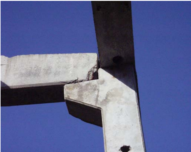
Figure 1.11 Concrete Spalling
