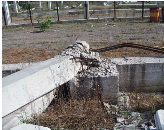
Figure 1.9 Damage Near the Base of Columns
