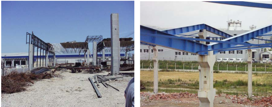
Figure 7.1 Industrial Buildings with Steel Trusses or Girders
