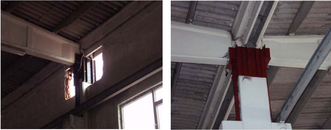
Figure 6.22 Steel Clamps Used to Retrofit Connections
